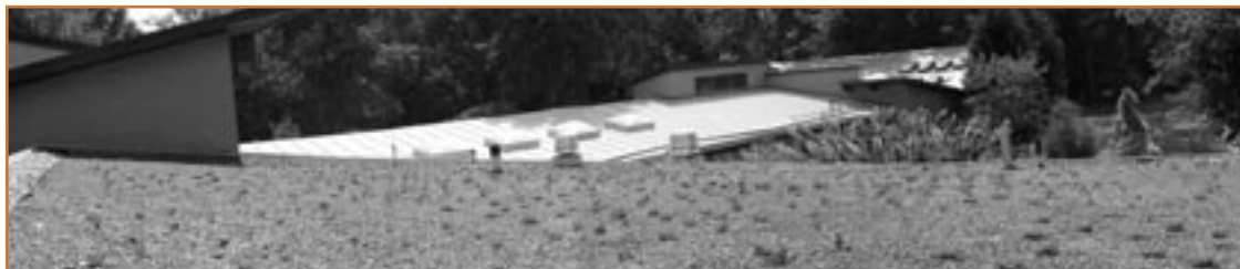
SCEE's new green roof, shown here in a panoramic view, will help conserve energy and decrease stormwater runoff.
